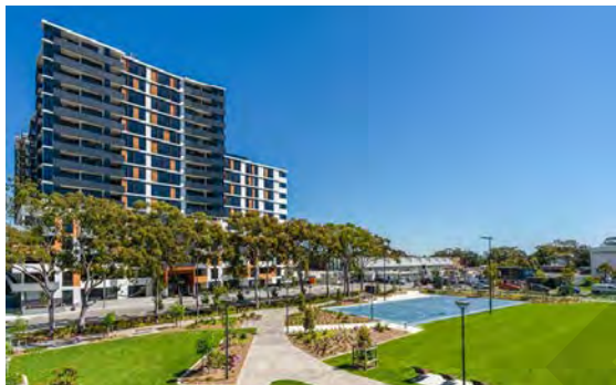
High densities of the Eastgardens development are located to the south-west of the subject site.
