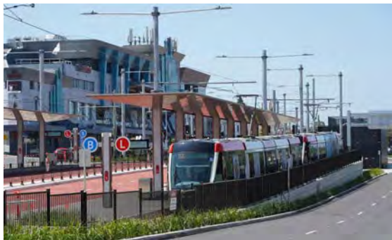
Kingsford Light Rail Terminal
